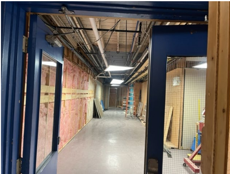
Figure 4 gym corridor being prepped for demolition
