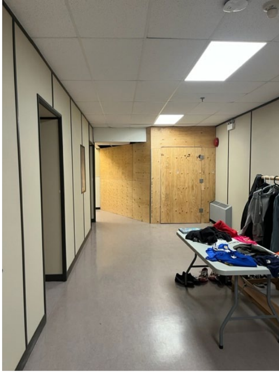
Figure 5 new hoarding for gym corridor
