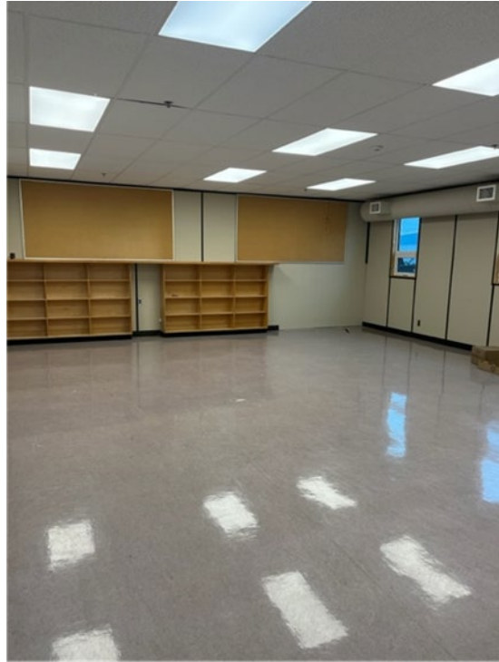
Figure 6 classroom moved out and ready for renovation
