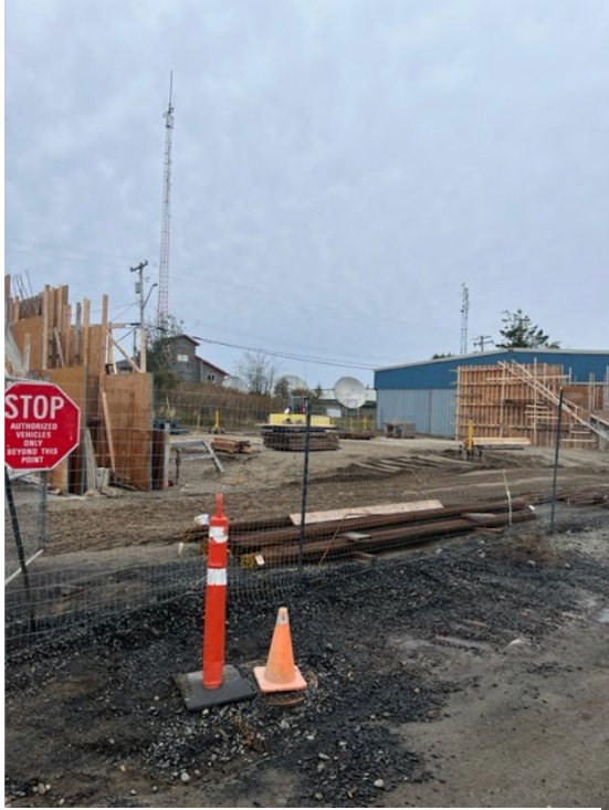
Figure 7 Tsunami tower stair walls poured
