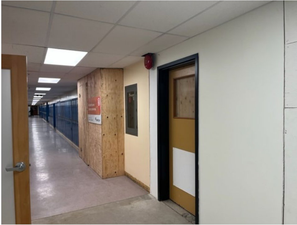
Figure 3 temporary lockers installed and hording to gym corridor installed
