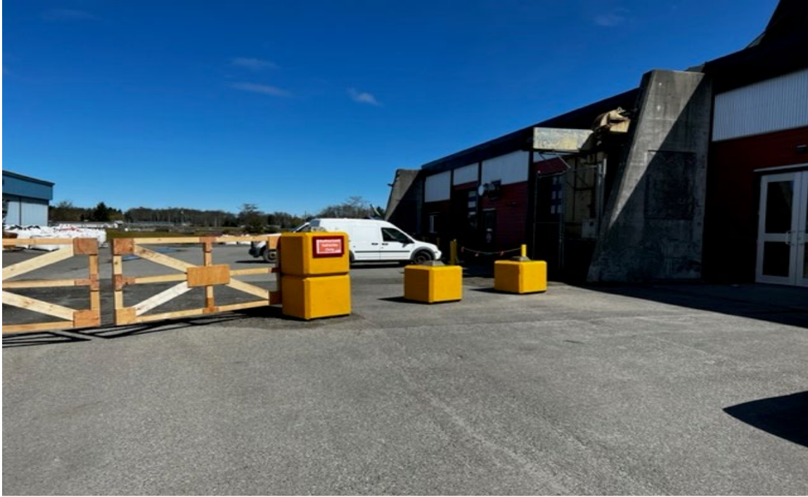
Figure 3 Construction gate to keep public traffic out of loading and unloading zone
