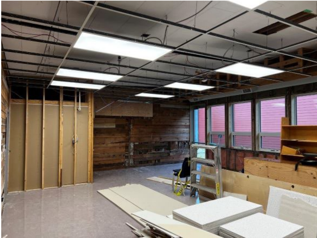
Figure 2: Classroom 30 just about ready for seismic upgrade.
