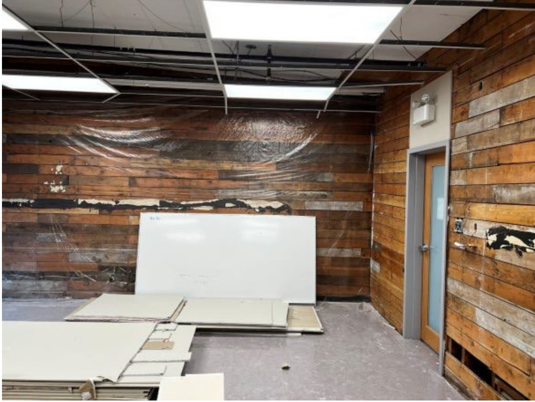
Figure 3: Classroom 31 nearly ready for seismic upgrade.
