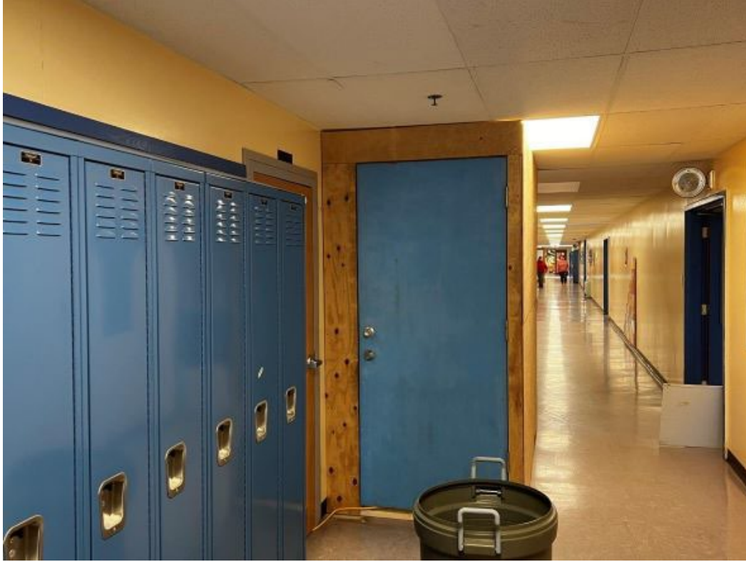
Figure 1: Hoarding of classroom while emergency exits being installed.
